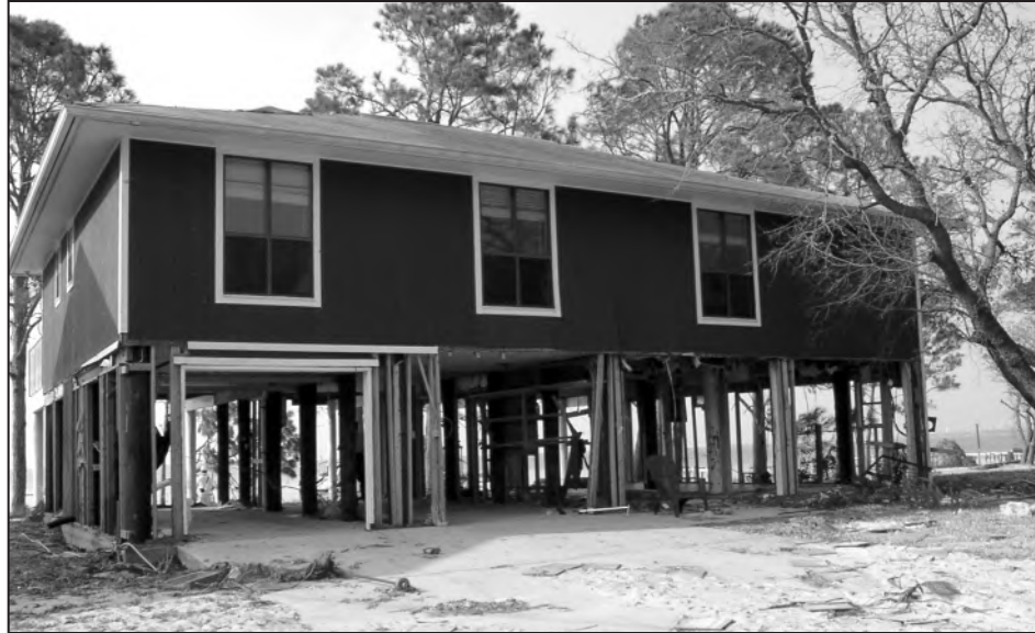
Figure 19. Structure elevated above BFE in AE zone showing successful response of breakaway walls
